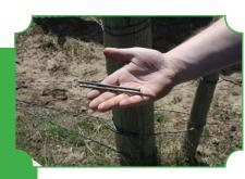
Using 24D pole barn nails, position the latch in place on top of the post.
