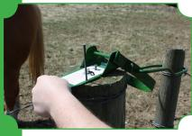
Start the top nails in, making sure to have the gate latch in the correct position
